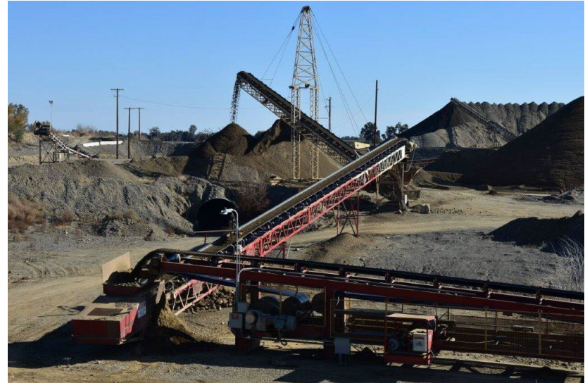
Aggregate Material Conveyed from Teichert Shifler
