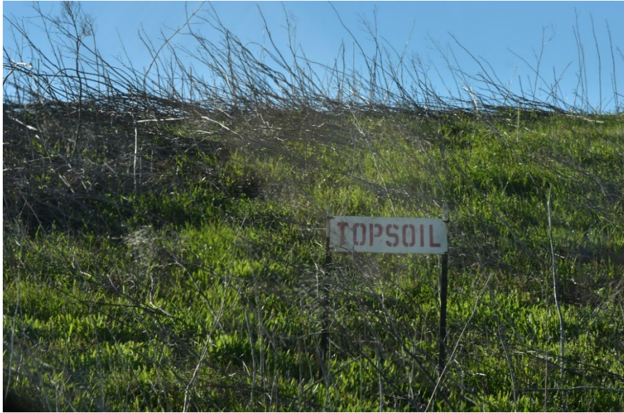
Vegetated Soil Stockpile with Signage
