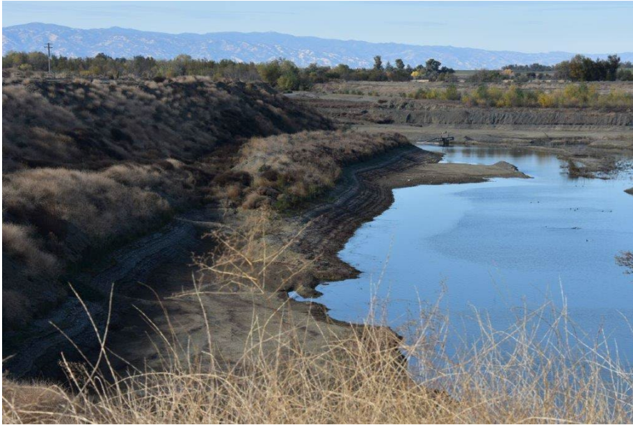
South Bank of Pit Looking West Additional Slope Grading needed for Reclamation
