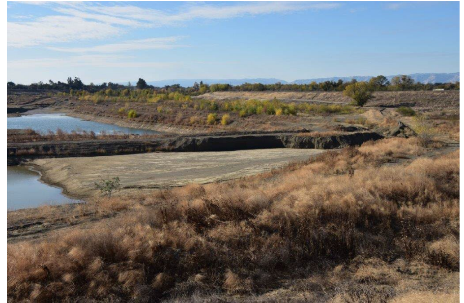
Soil Fill Area - Preparation for Reclamation
