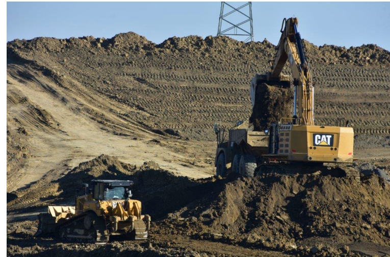
Overburden Removal 20-Acre Interim Mining Area
