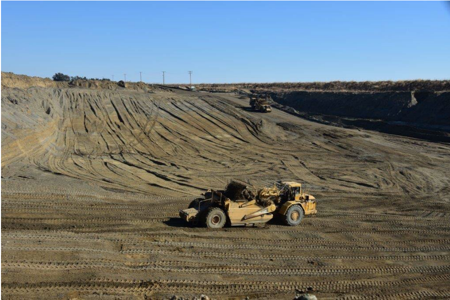
Shifler Aggregate Excavation using Scraper
