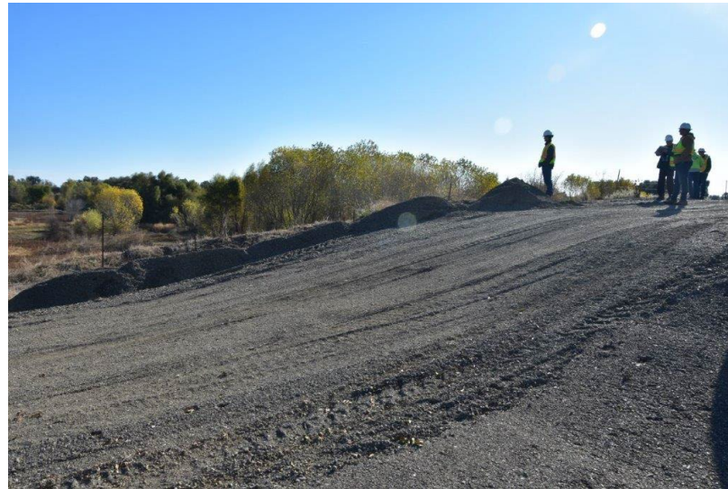
CR 96 Regrade – Access to Levee Road Looking Southeast
