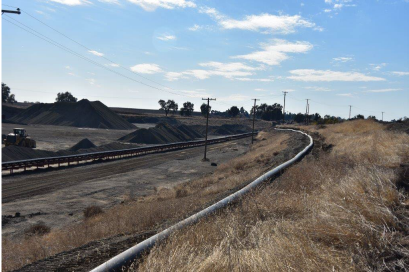
Conveyor from Teichert Shifler to Woodland Plant
