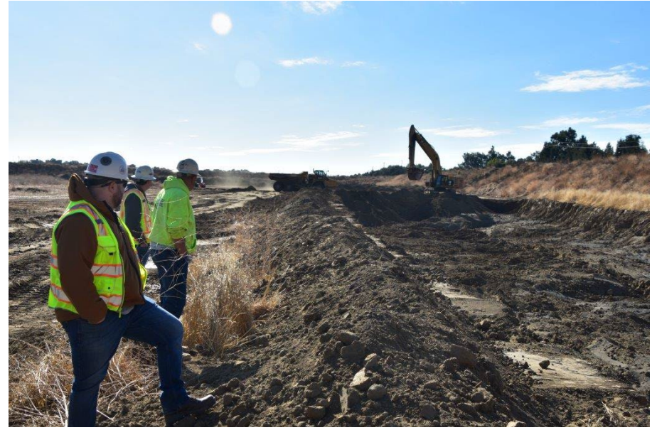
Overburden Removal using Excavator
