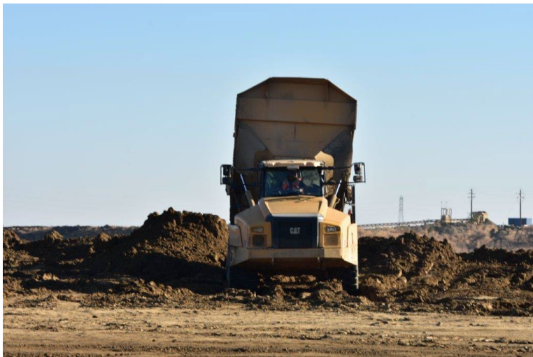
Depositing Overburden Soil for Future Reclamation
