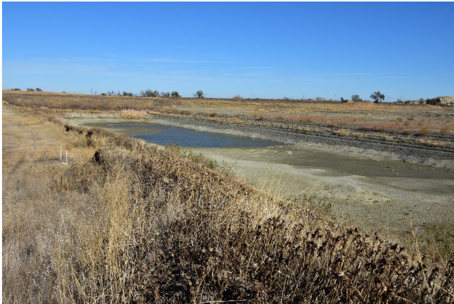
Previously Mined Area A2 – 2022 Inspection
