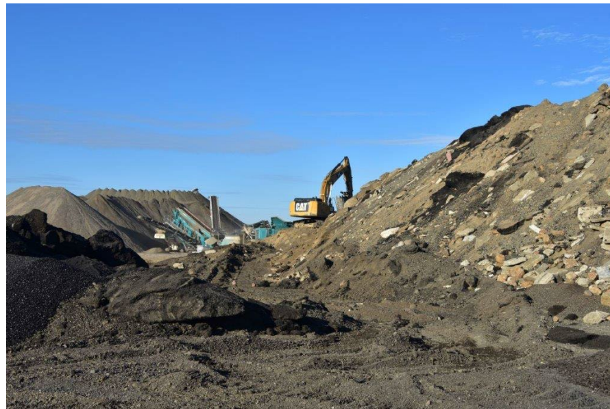
Concrete Recycling Teichert Woodland Plant
