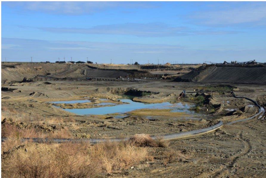
Wash Fines Pumped into Pit for Future Reclamation
