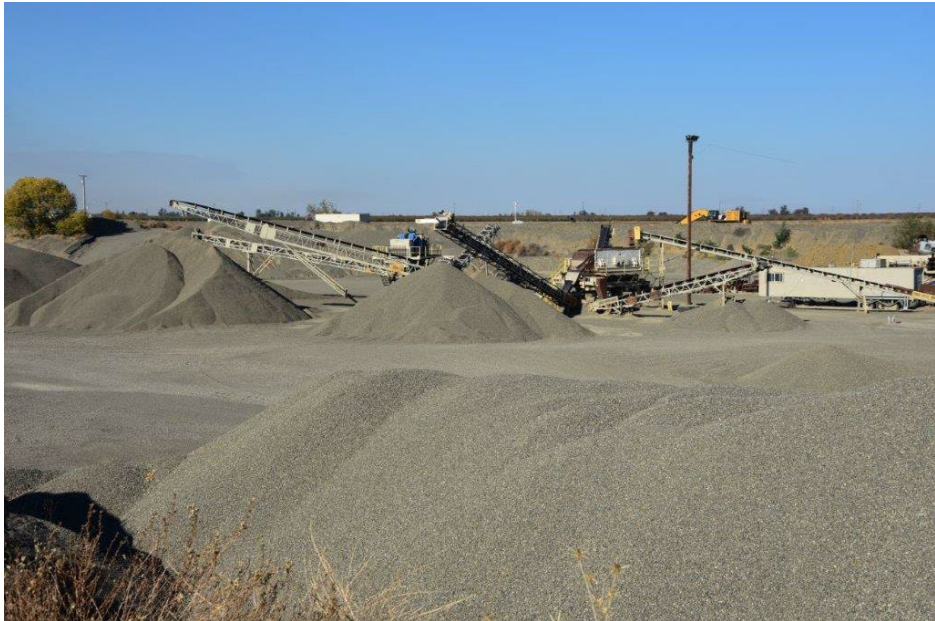
Esparto Plant & Stockpiles Looking North
