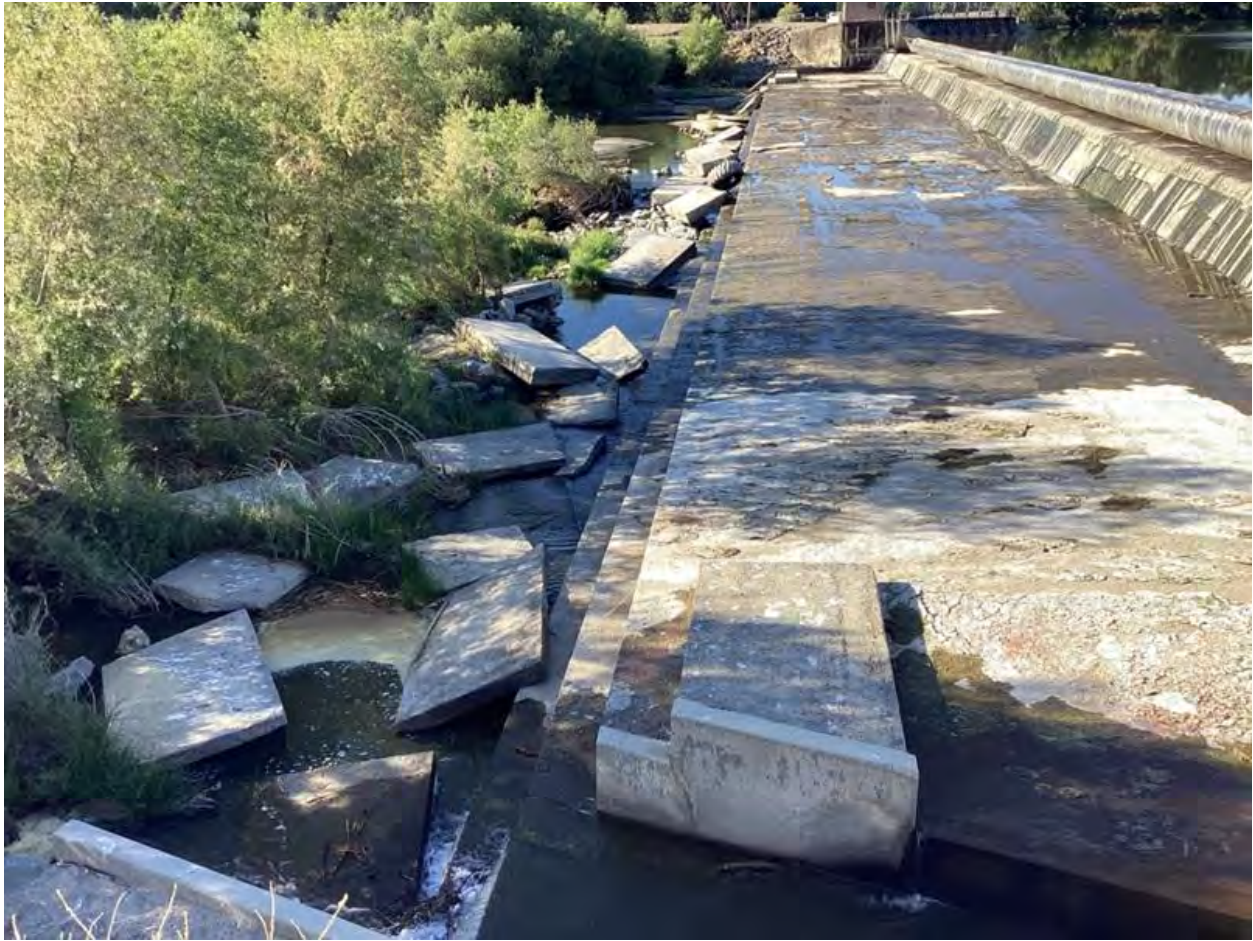
Figure 2-13. Capay Dam and apron. (2024)
