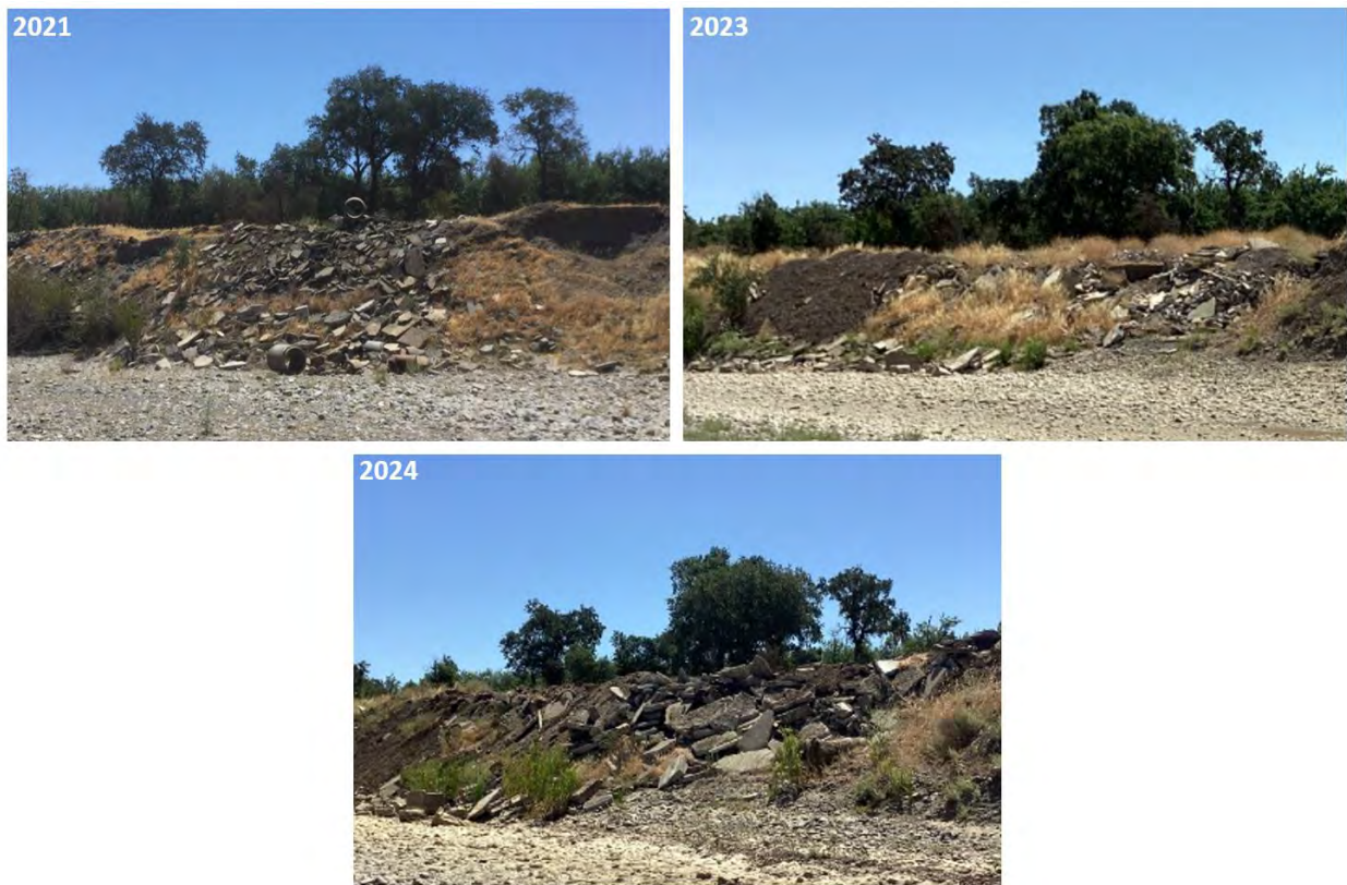
Figure 2-18. South (right) bank at River Mile 25.4 showing installation of concrete rubble in 2021, addition of new soil fill in 2023, and addition of new rubble in 2024.
