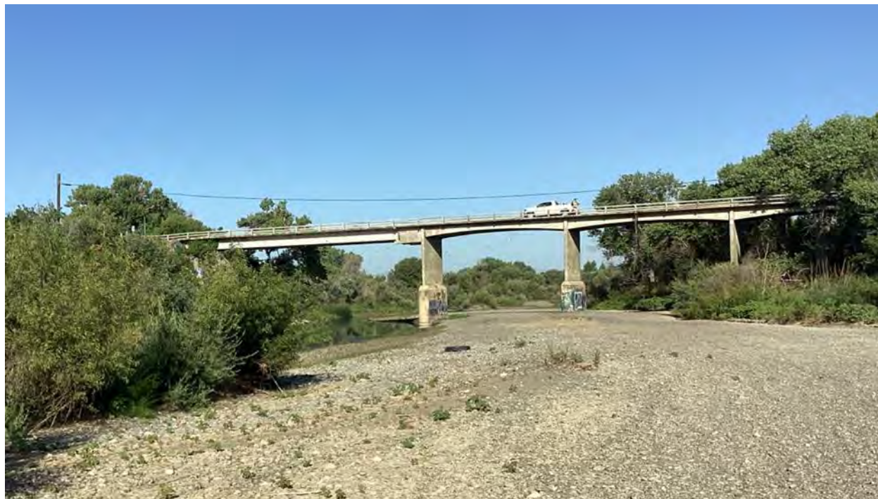
Figure 2-24. Looking upstream at the Stephen's Bridge (County Road 94B). (2024)
