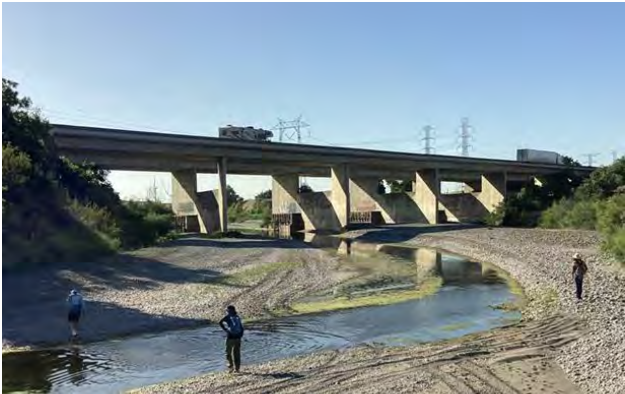
Figure 2-23. Looking upstream at I-505 Bridge. (2024)
