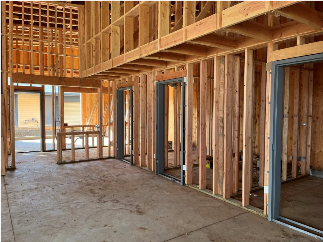
Image 02 – Building J Digital Media Classroom
