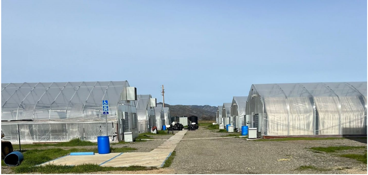
Site conditions in 2022 (submitted by applicant as part of application submittal)
