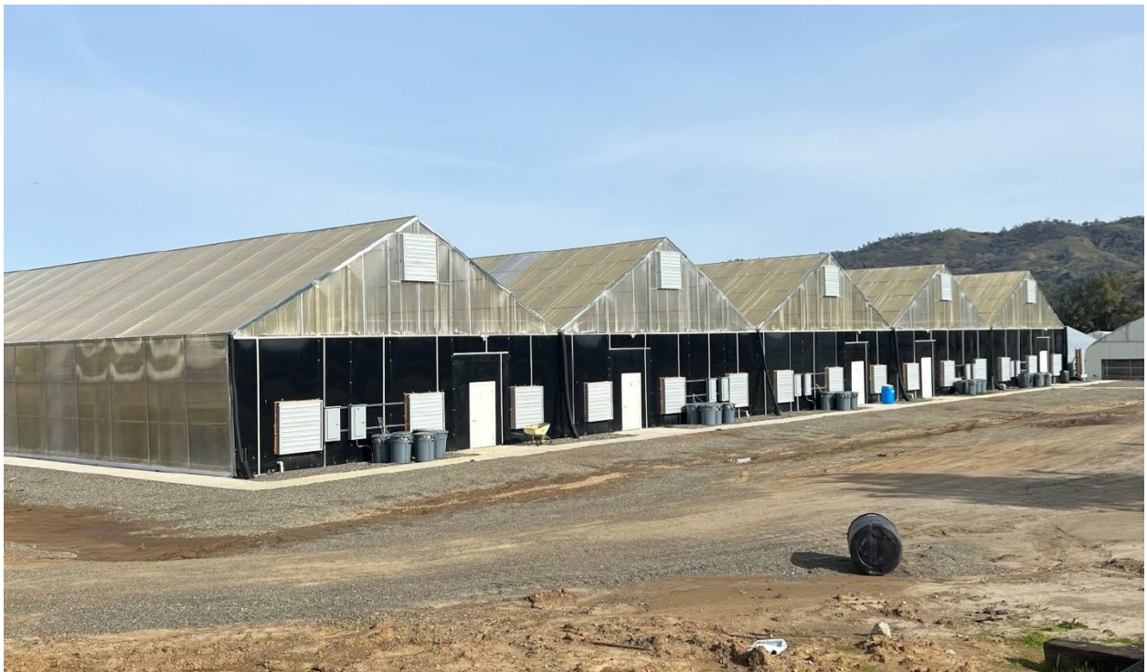
Site conditions in 2022 (submitted by applicant as part of application submittal)
