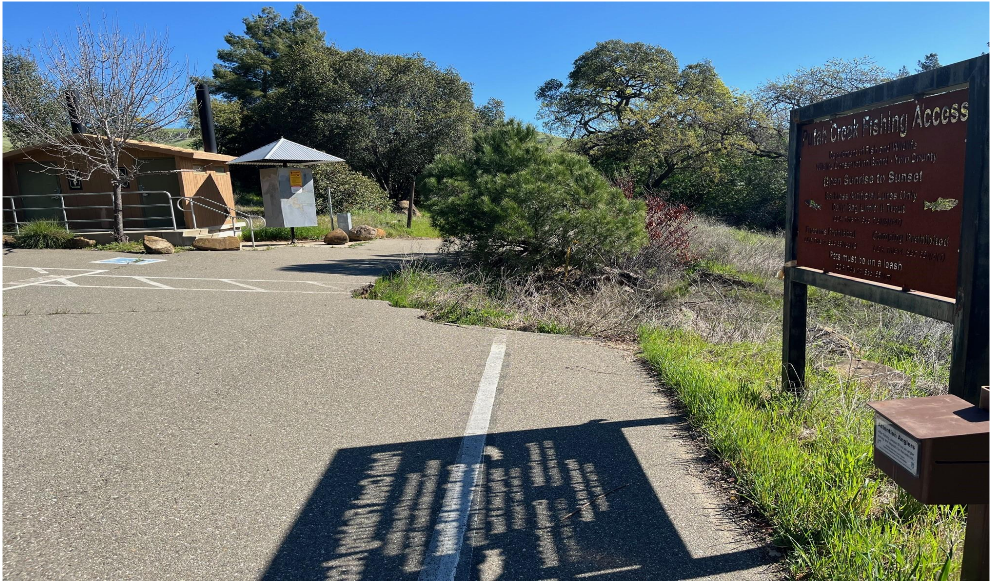
Site 3 West: Currently Closed due to erosion of parking lot; Restroom, Interpretive Panels, Trail
