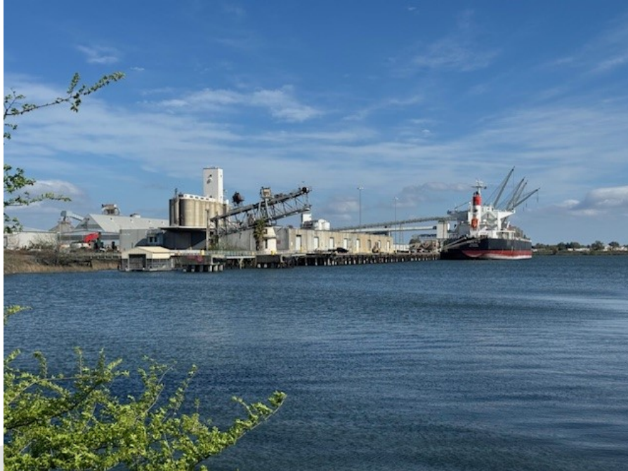
View of Port Across Lake Washington
