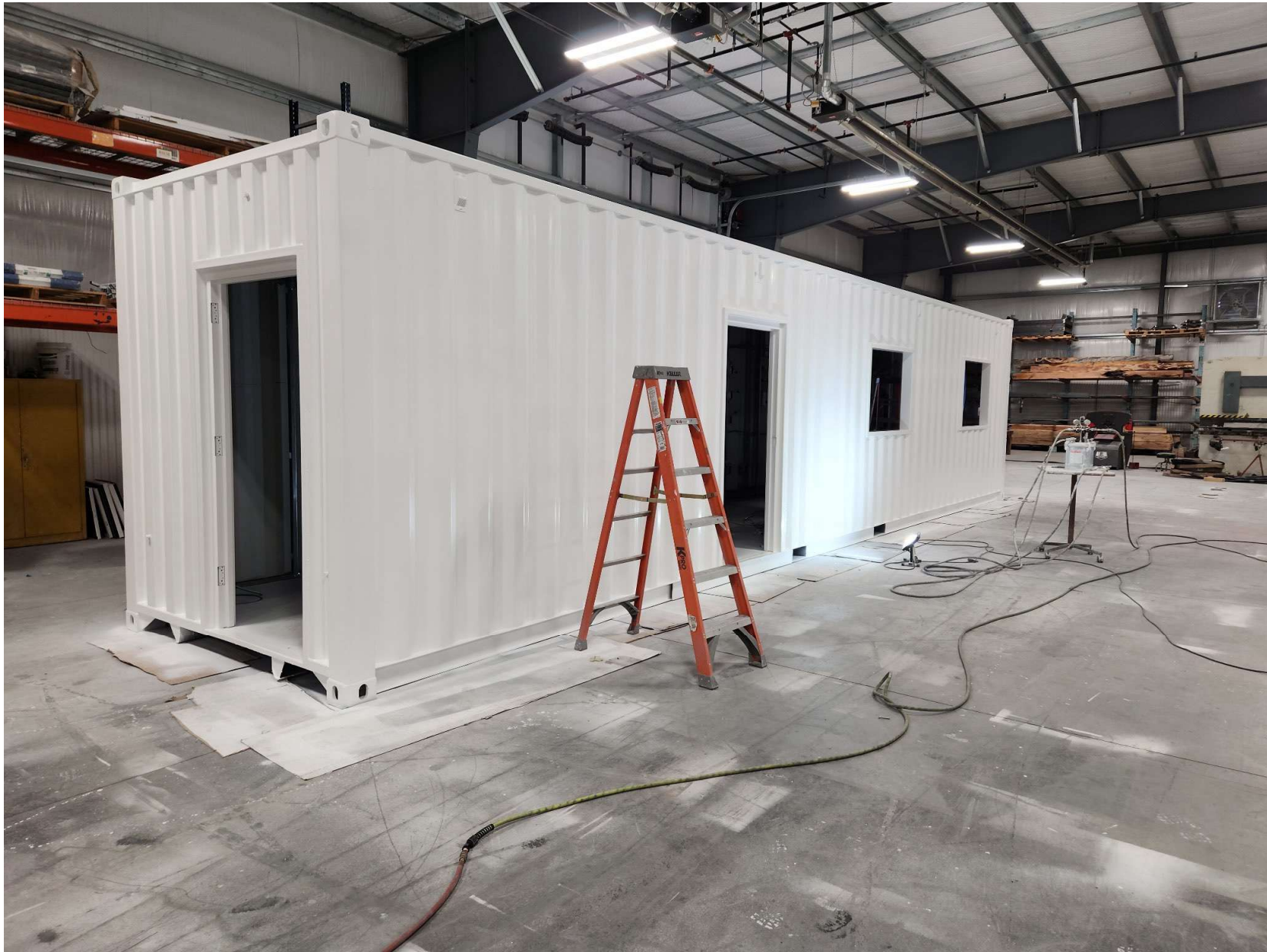
EXTERIOR CONSTRUCTION YCAS-CIAC
