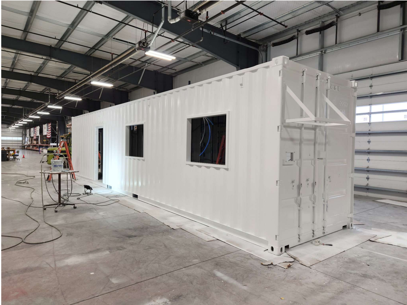
EXTERIOR CONSTRUCTION YCAS-CIAC
