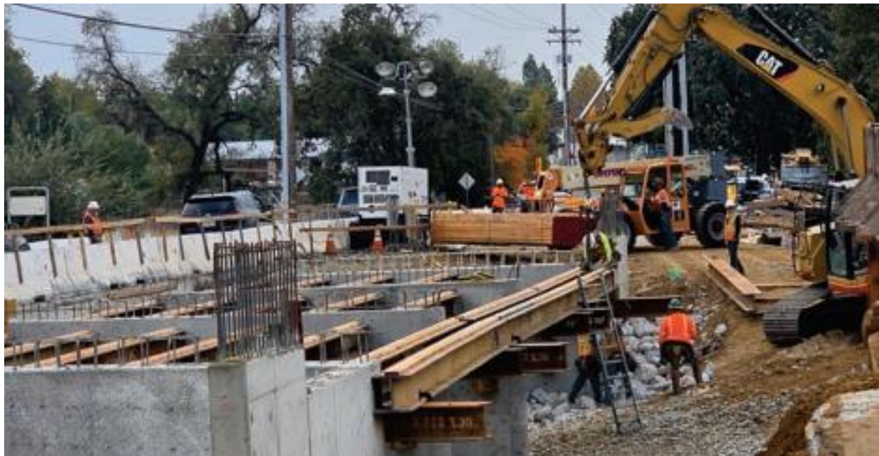
Eastside Road Bridge over Olney Creek in Redding
