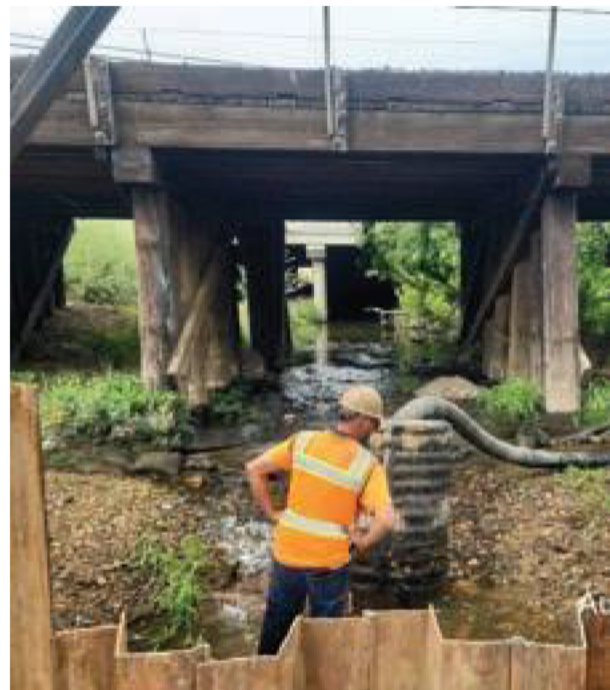
Temporary Creek Diversion System Eastside Road Bridge
