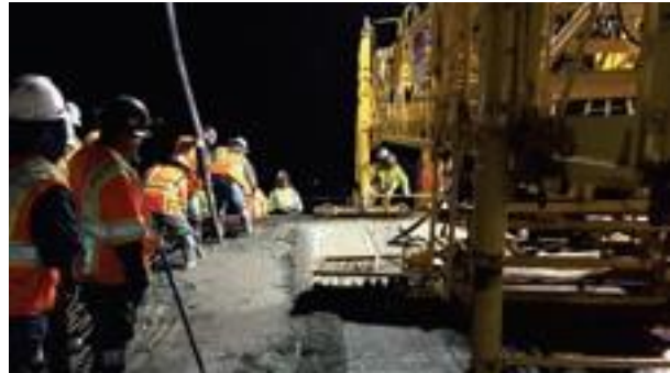
Dry run of Bidwell is critical for a quality deck finish
